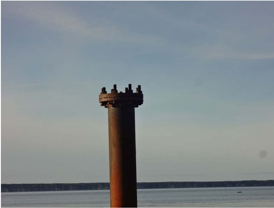
Photo 2 – Cap Casing of Well Repair #1
