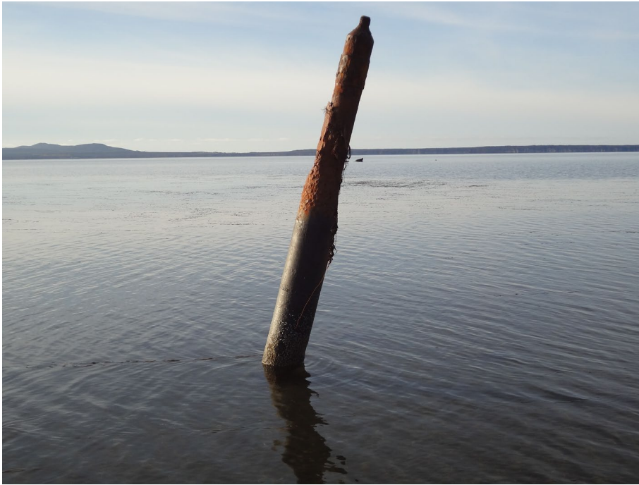
Photo 4 – Abandoned Oil Well Casing
