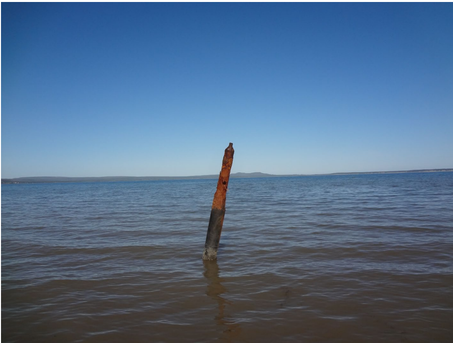
Photo 3 – Abandoned Well Casing
