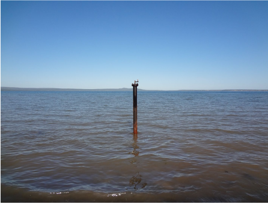
Photo 2 – Extension Pipe of Well Repair #1
