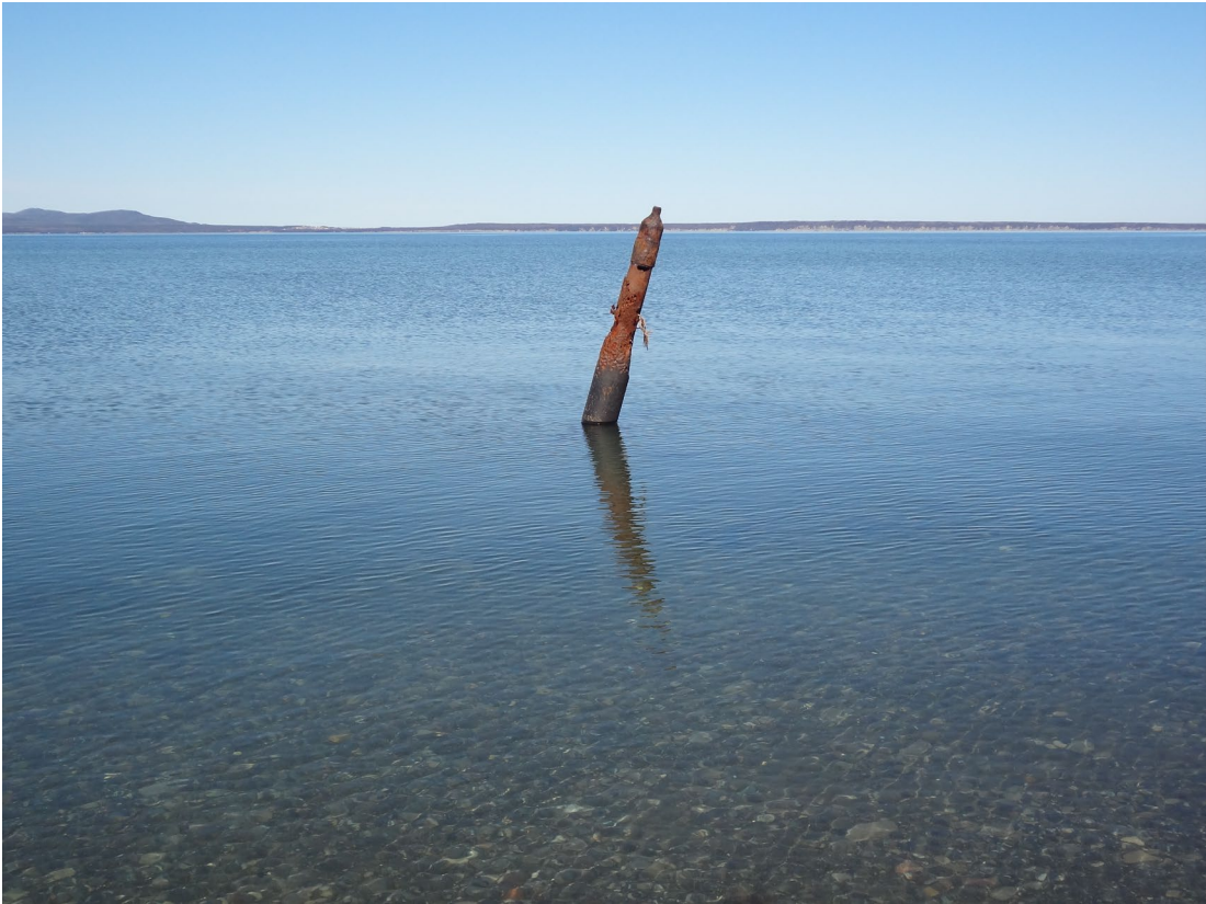
Photo 2 – Abandoned Oil Well Casing (Closest to the Shoal Point Tip)
