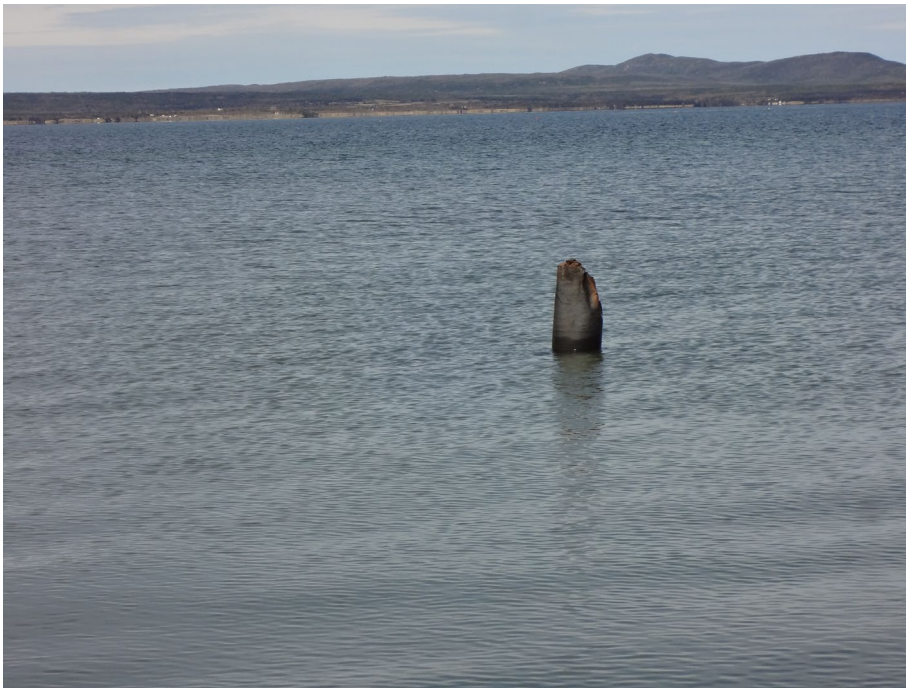
Photo 3 – Abandoned Oil Well Casing (Furthest from the Shoal Point Tip)
