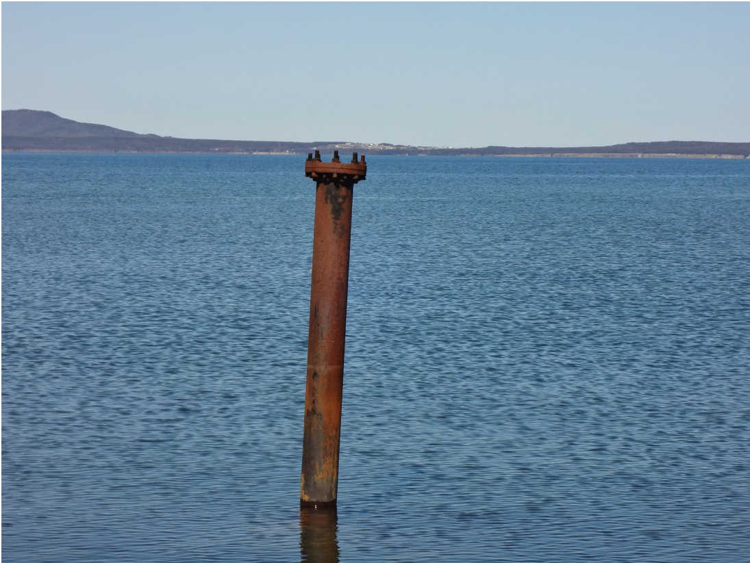
Photo 1 – Abandoned Well Repair #1
