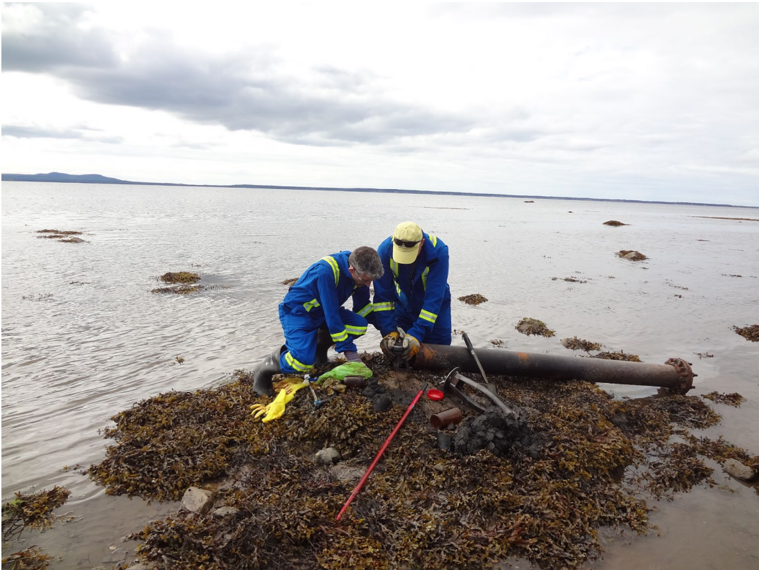
Photo 1 – Plug Installation Well #1
