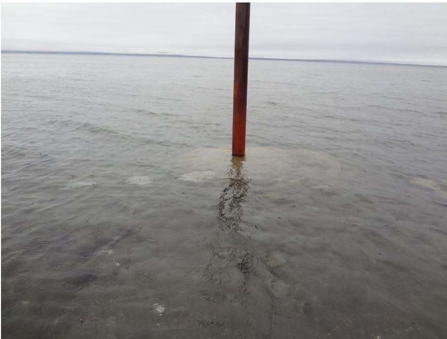
Photo 3 – Visible oil in vicinity of Well Repair #1
