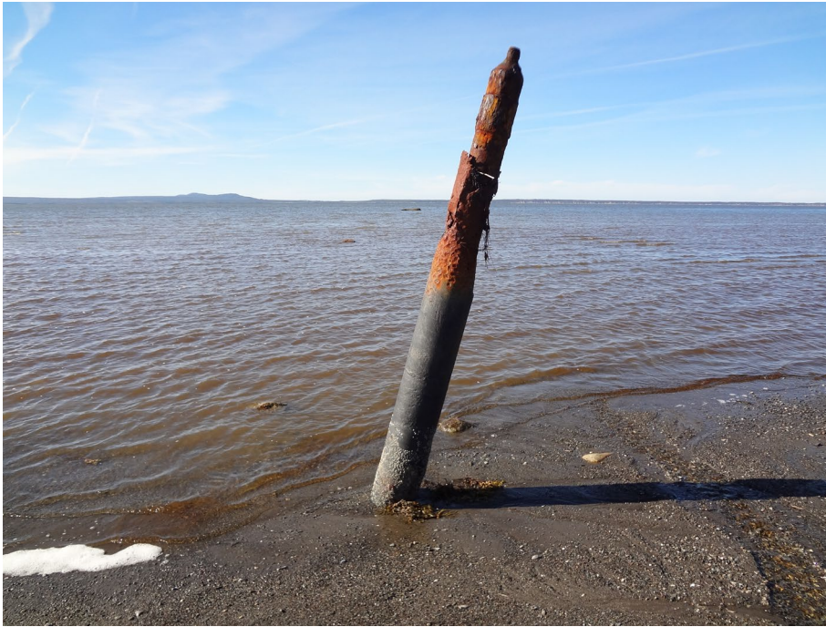
Photo 4 - Abandoned Well Casing
