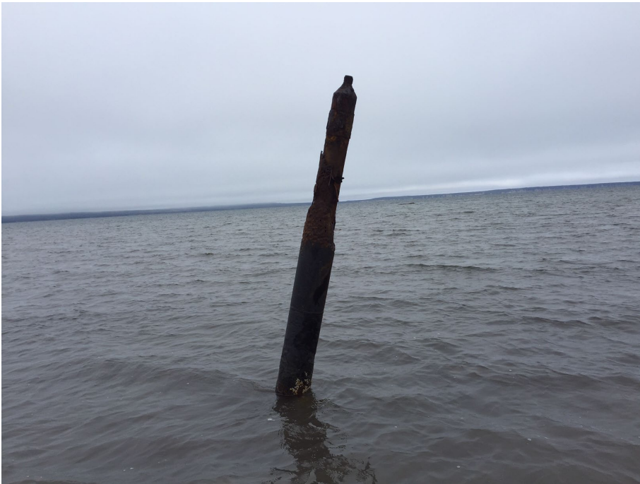
Photo 5 – Abandoned Well Casing
