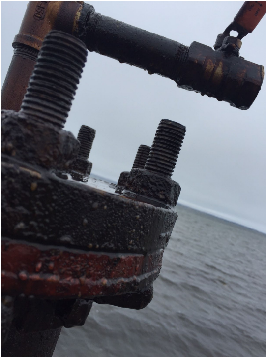
Photo 2 – Top of Extension Pipe of Well Repair #1
