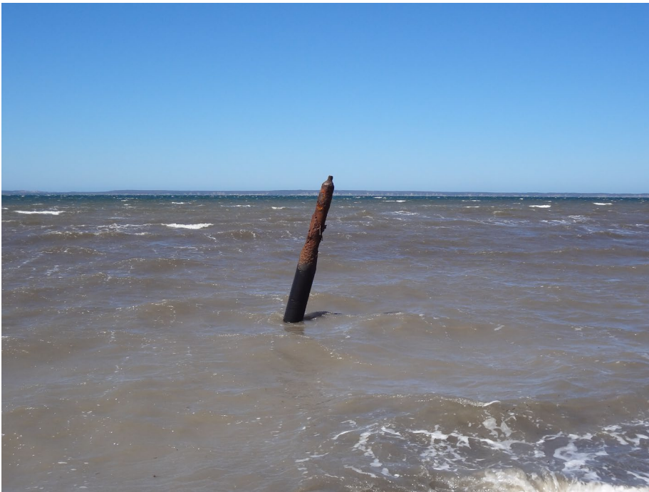
Photo 3 - Abandoned Well Casing
