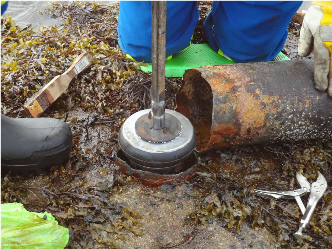
Photo 2 – Plug Installation Well #1
