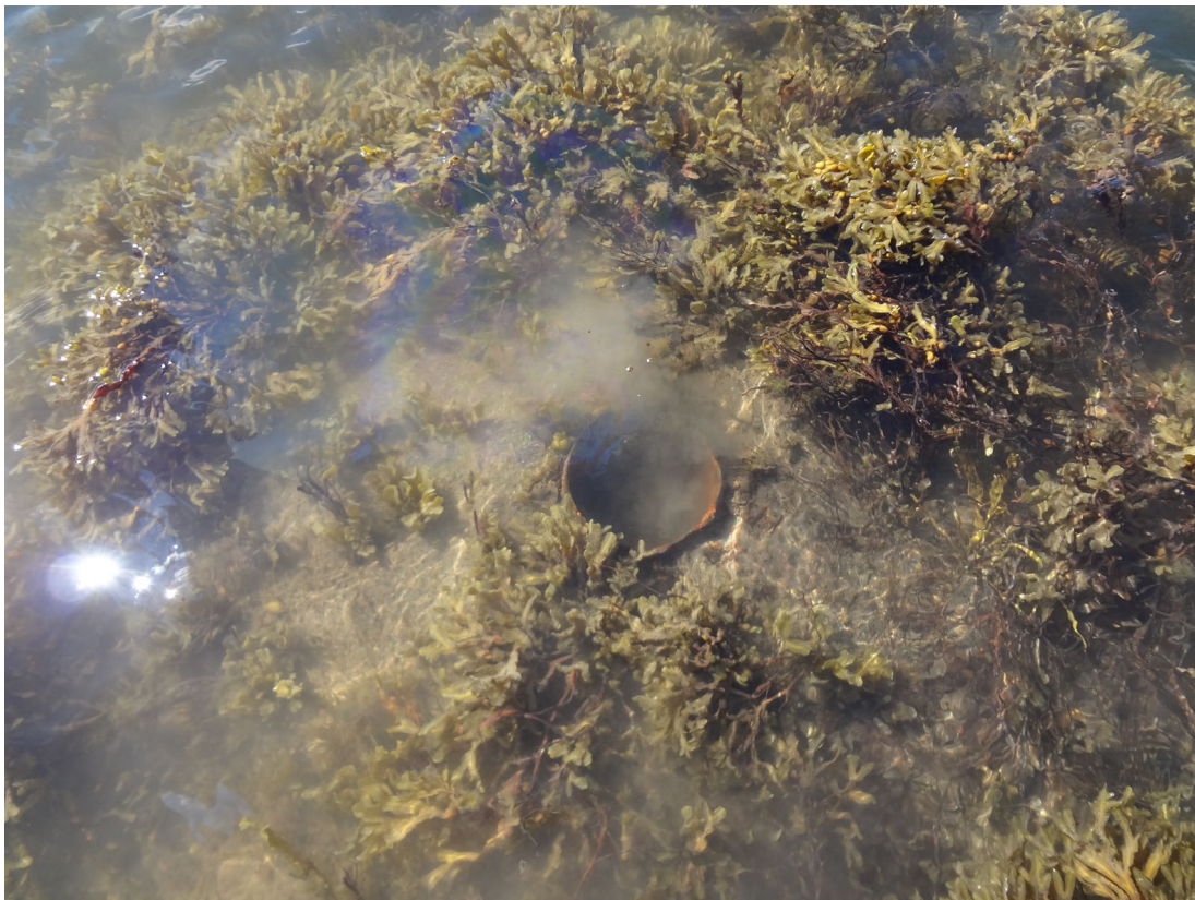
Photo 3 – Oil sheening and Bubbles at Well #1 (Cap Removed)
