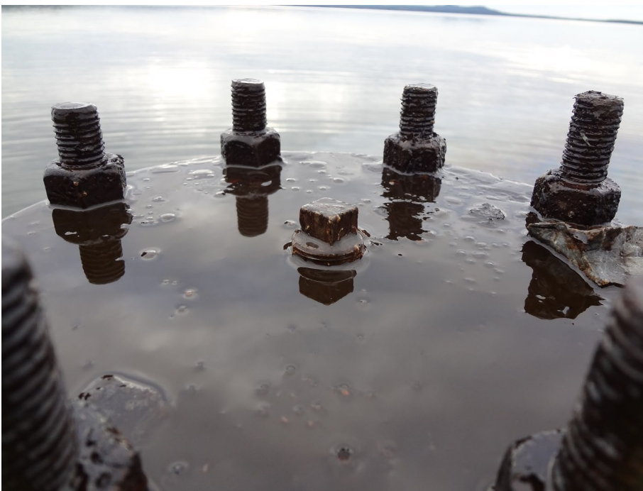
Photo 3 – Threaded Fitting in Top Plate of Well Repair #1
