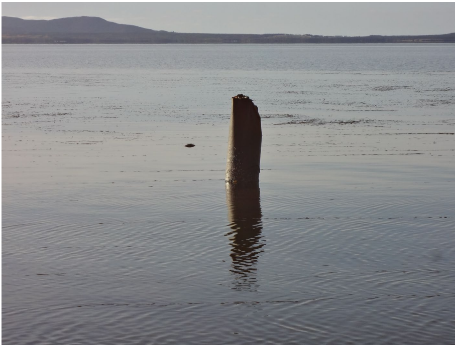
Photo 3 – Abandoned Oil Well Casing
