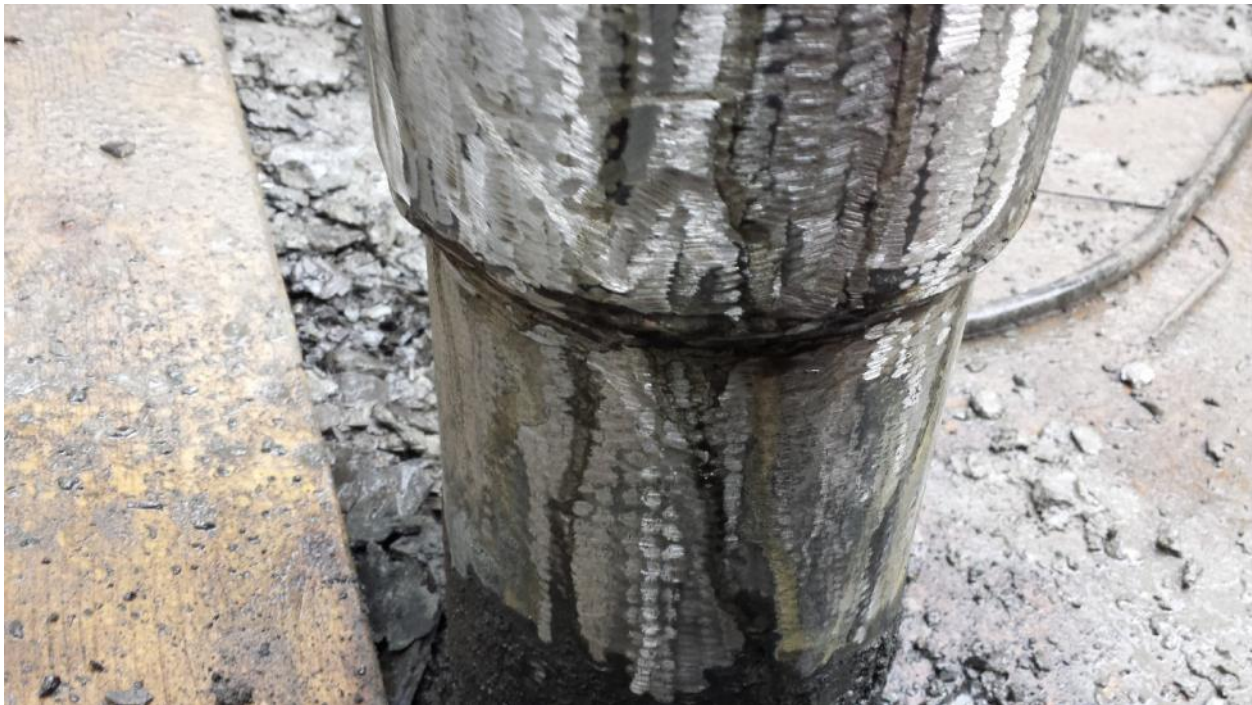
New 6" ID riser pipe welded onto old 6" OD casing (5" overlap)
