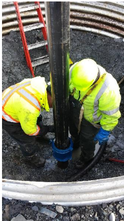
Photo 4 – Workers installing 150 mm \varnothing pipe extension.
