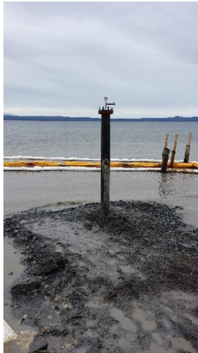
Photo 1 – View of completed well casing extension (Well Casing No. 1).
