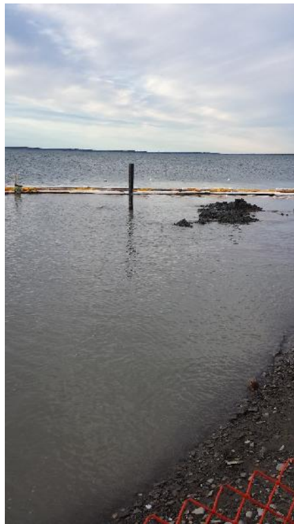
Photo 8 – Well casing No. 1 completed.
