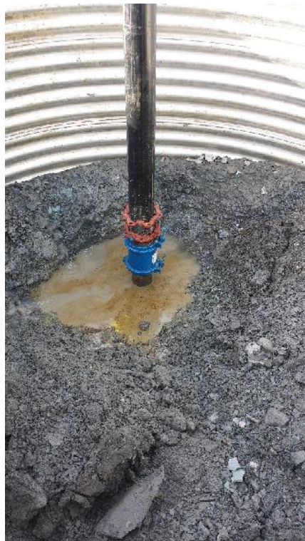
Photo 6 – Megalugs installed at base of new pipe extension.
