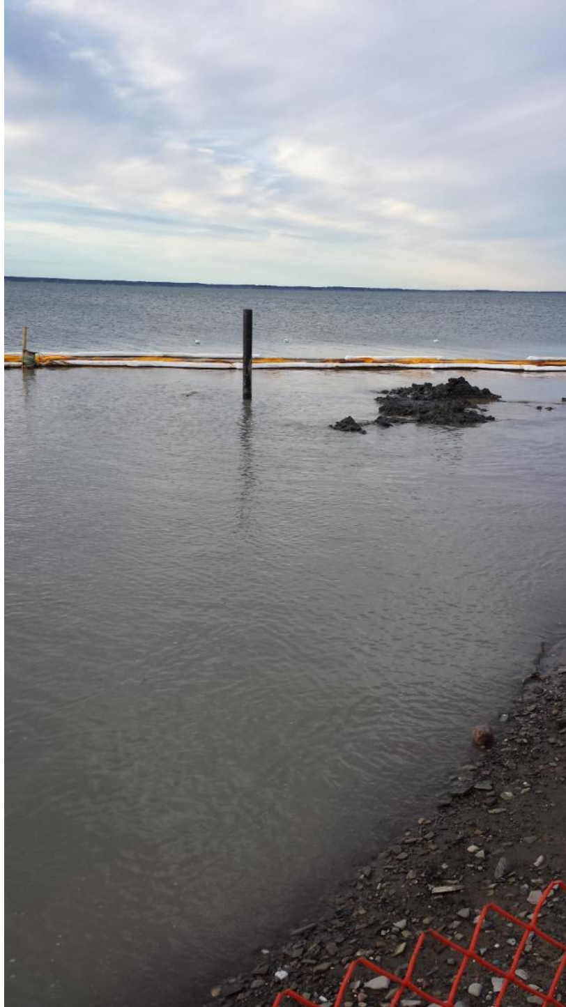
Riser in Place and Culvert Removed
