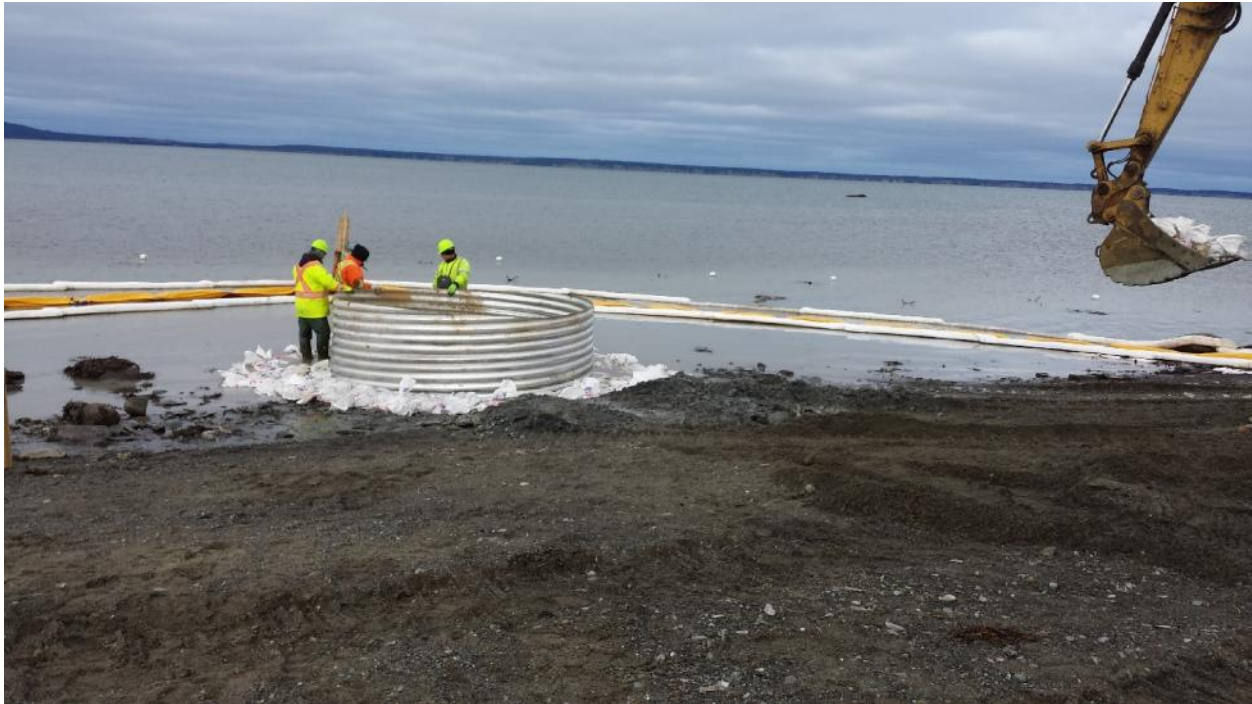
Placing of Sand Bags Around Culvert at Low Tide About 10 AM
