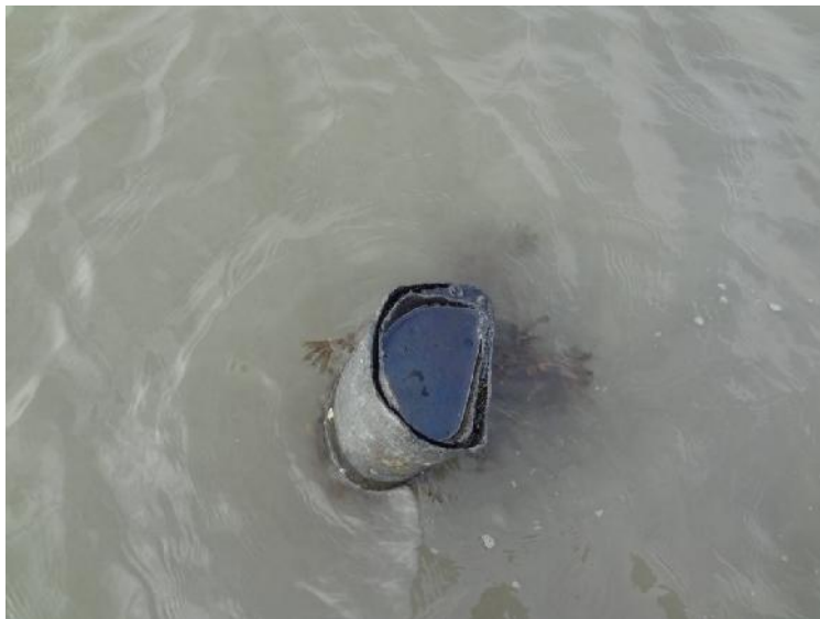
Photo 8 – Close-up view of leaking oil well casing No. 2 to the south of the main well casing.
