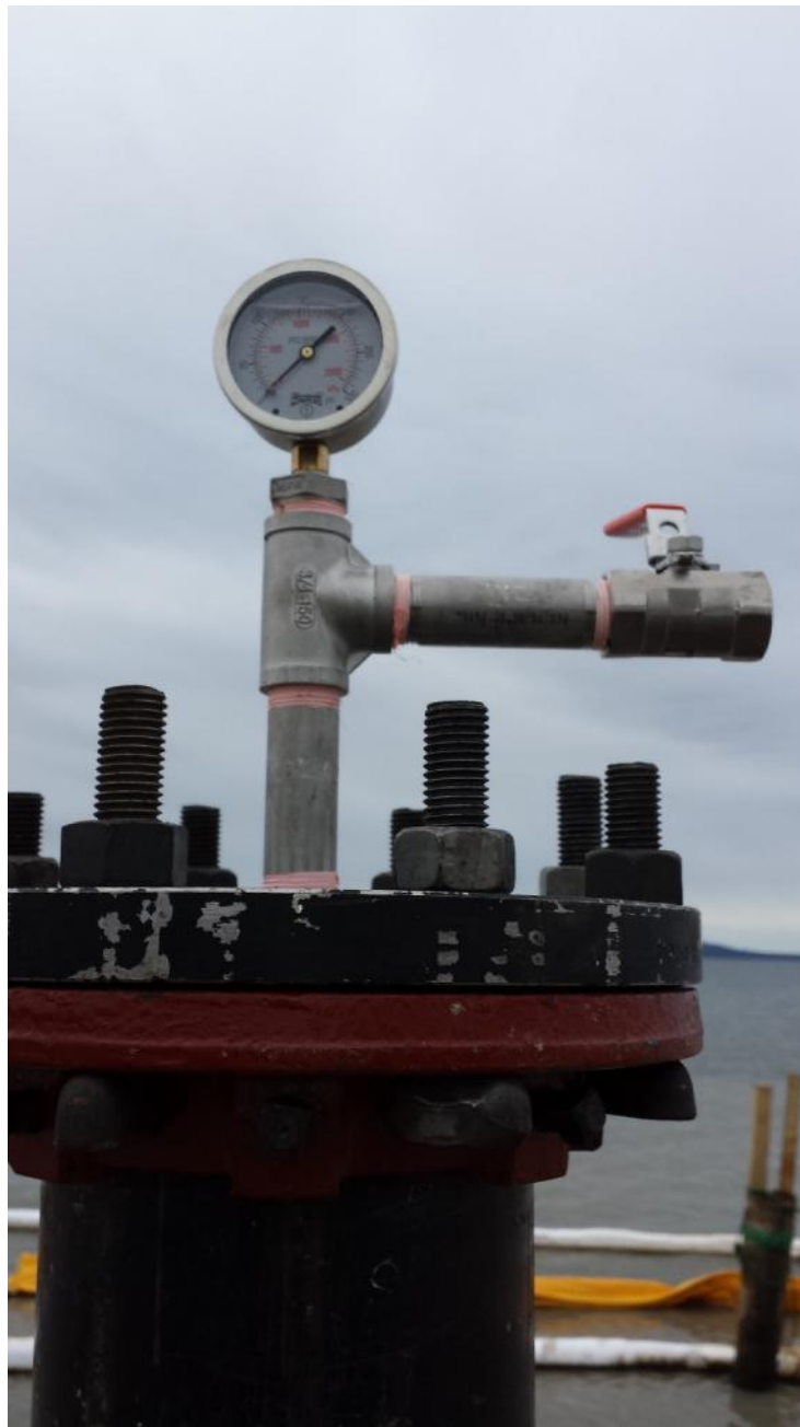
Final Installation of Flange and Fittings
