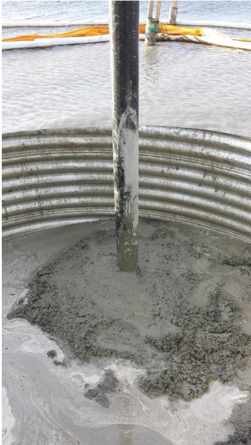
35 MPa concrete placed
