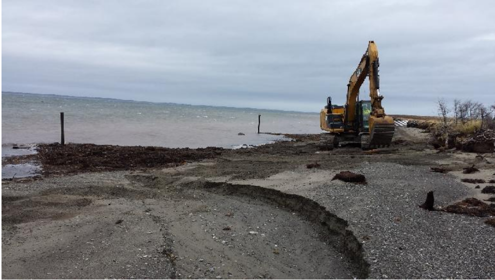
Photo 1 – Excavator cleaning up and demobilizing from site.
