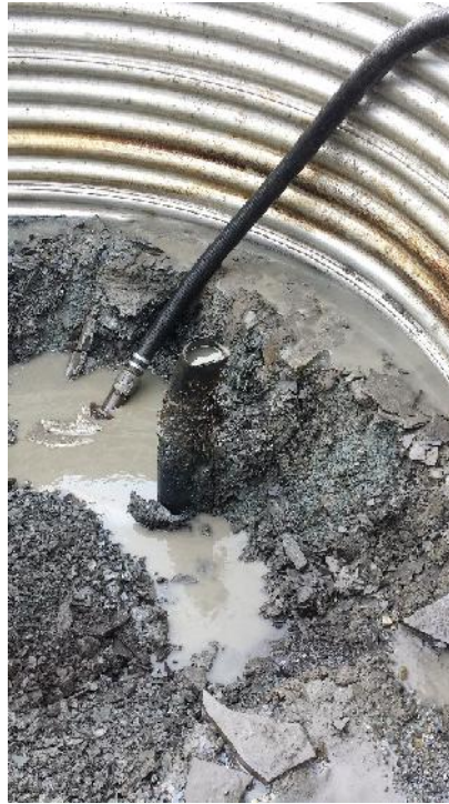
Photo 1 – View of exposed well casing No. 2
