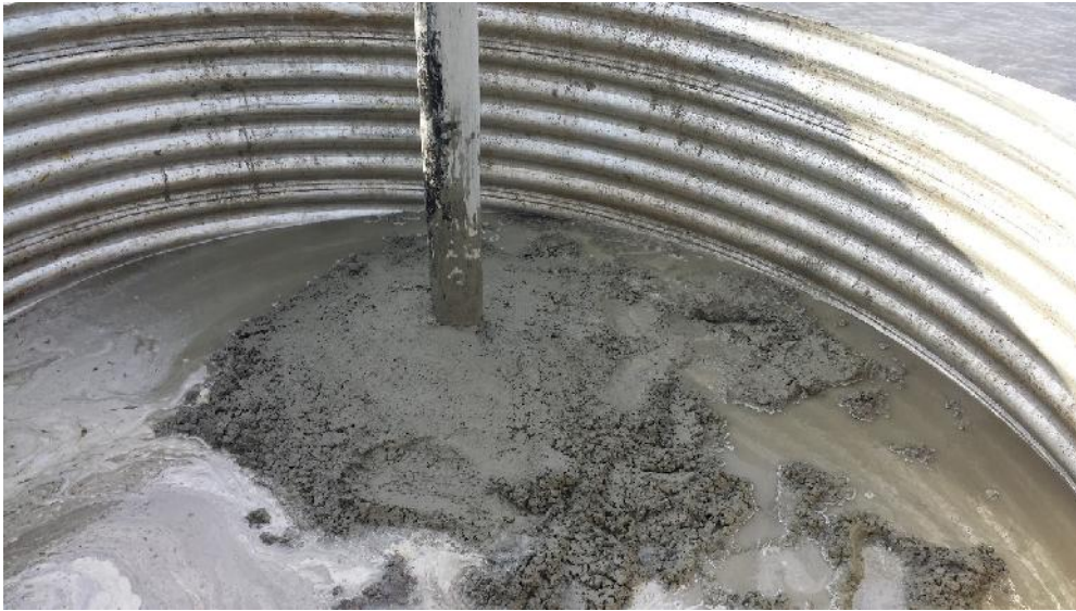
Photo 7 – Concrete fill placed around coupling and megalugs.
