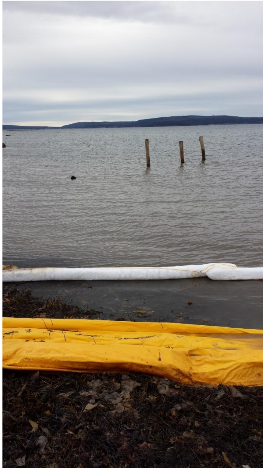
Well #2 with posts used to stabilize Oil Booms and Turbidity Curtain
