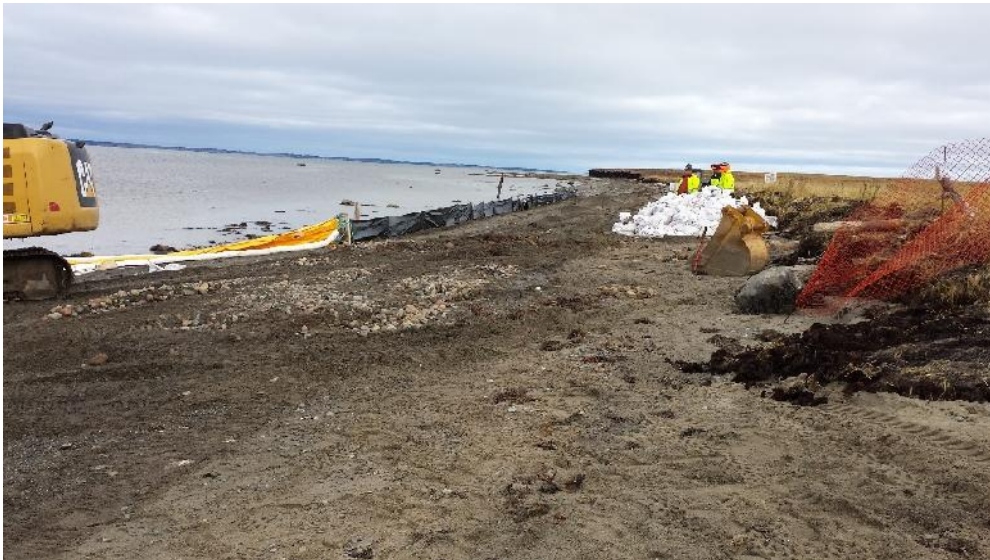
Photo 2 - View of silt fence in position along beach access.
