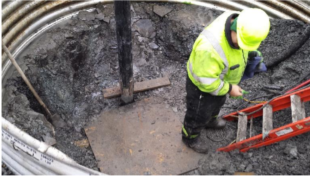
Photo 5 – View of completed extension pipe connection to existing casing.
