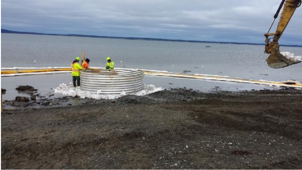
Photo 1 – Contractor installing culvert and sand bags at well casing No. 1 location.
