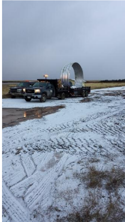
Photo 1 – Arrival of culvert at site in Shoal Point.
