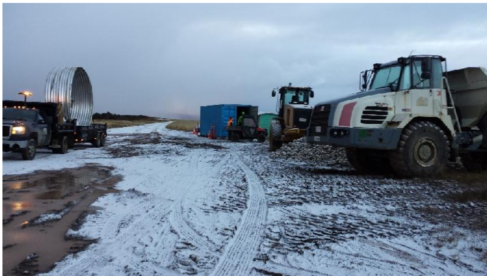
Photo 2 – View of mobilized contractor equipment at the lay down area.
