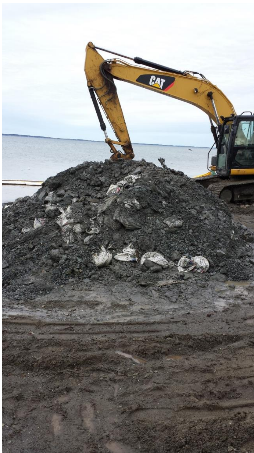
Contaminated Soil that was sent to the Remediation Center
