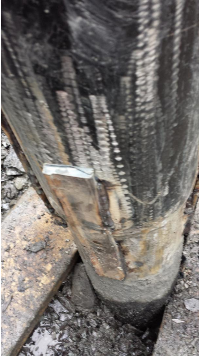
Welded on strap
