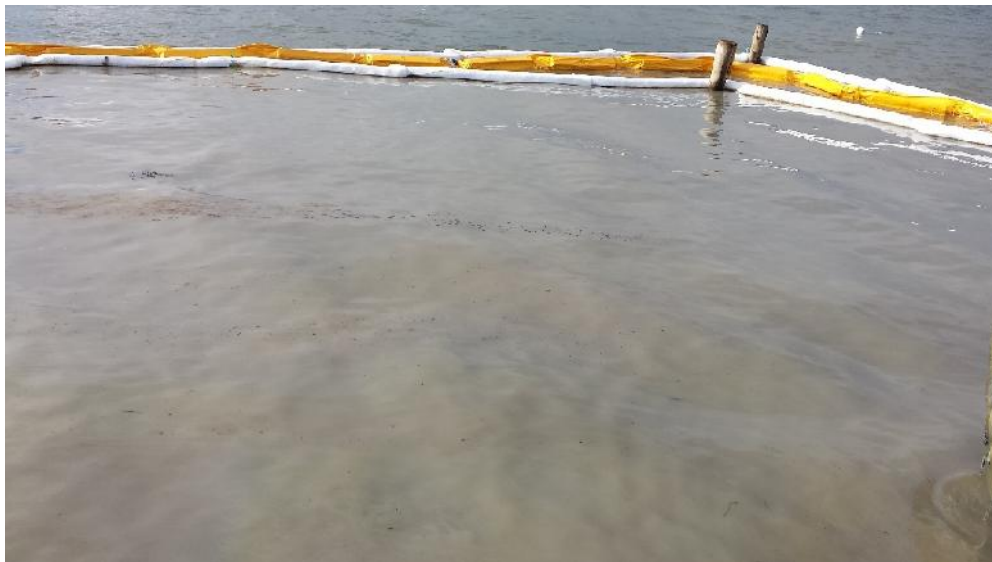
Photo 6 – Oil booms and turbidity curtain installed and anchored in position.
