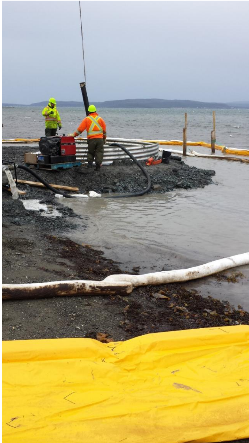
Work setup and lowering new riser
