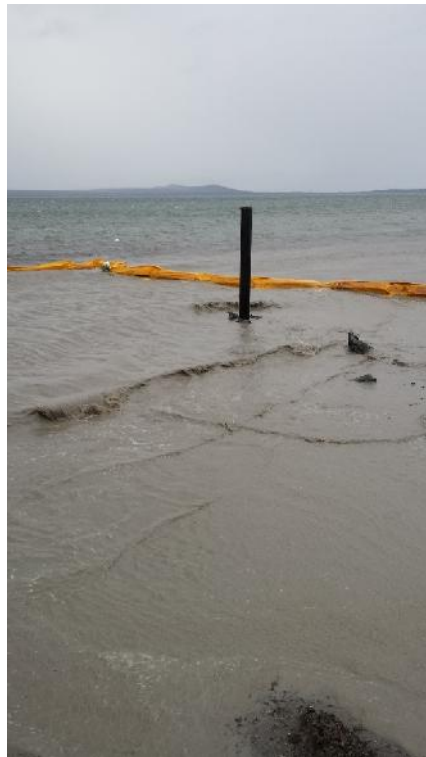
Photo 6 – View of completed well casing No. 2 prior to installation of pressure gauge and lockable outlet valve.
