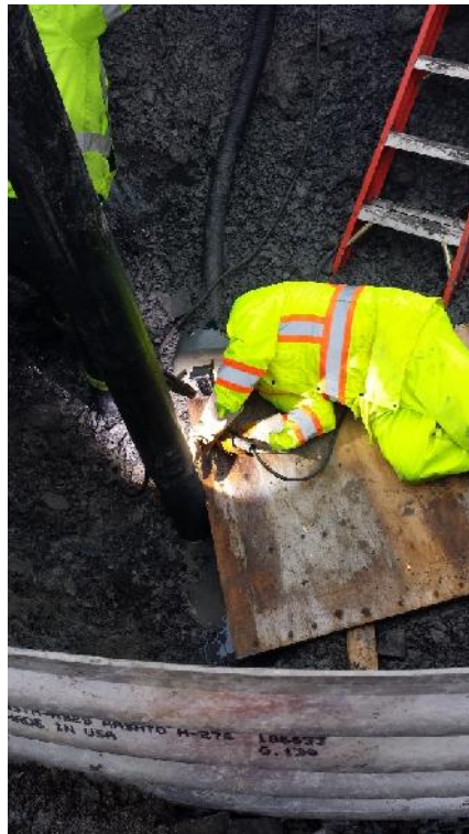
Photo 4 – Worker welding extension pipe onto existing well casing No. 2.
