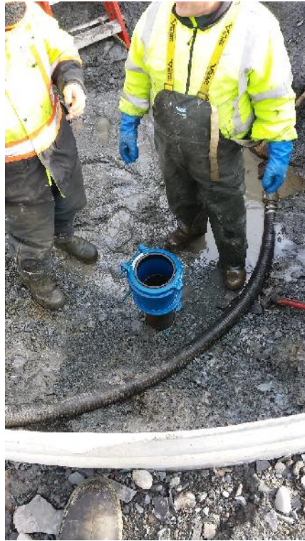
Photo 3 – Well casing No. 1 with adapter coupling in position.
