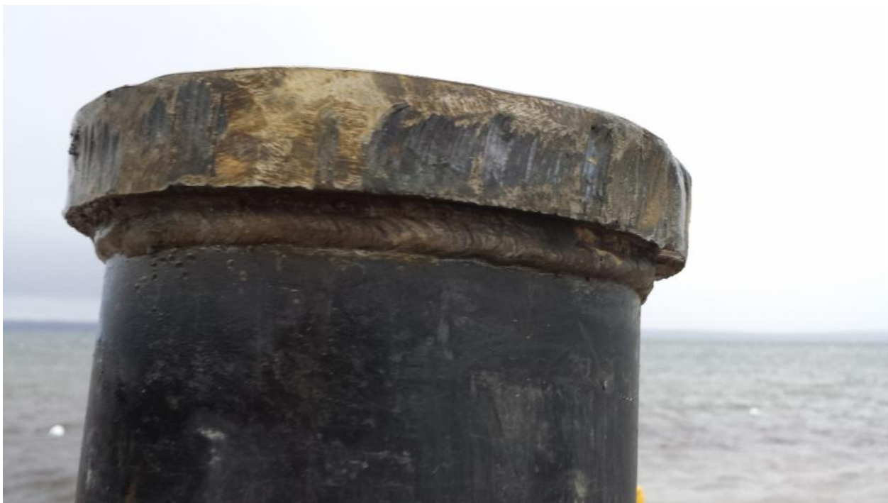
Modified 200 mm flange welded to Well #2 Riser
