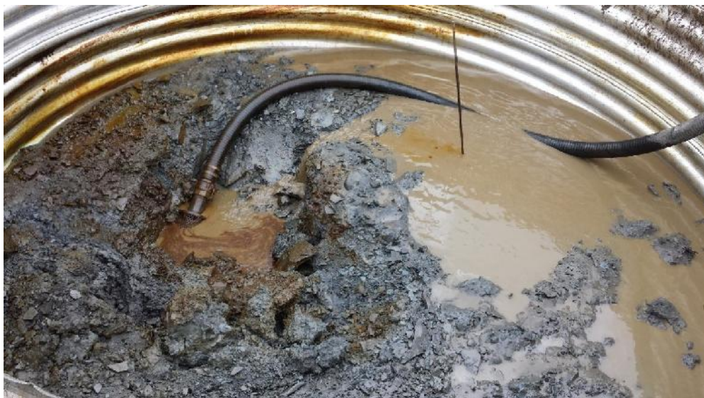
Photo 4 – Pumping the water out of the installed culvert.
