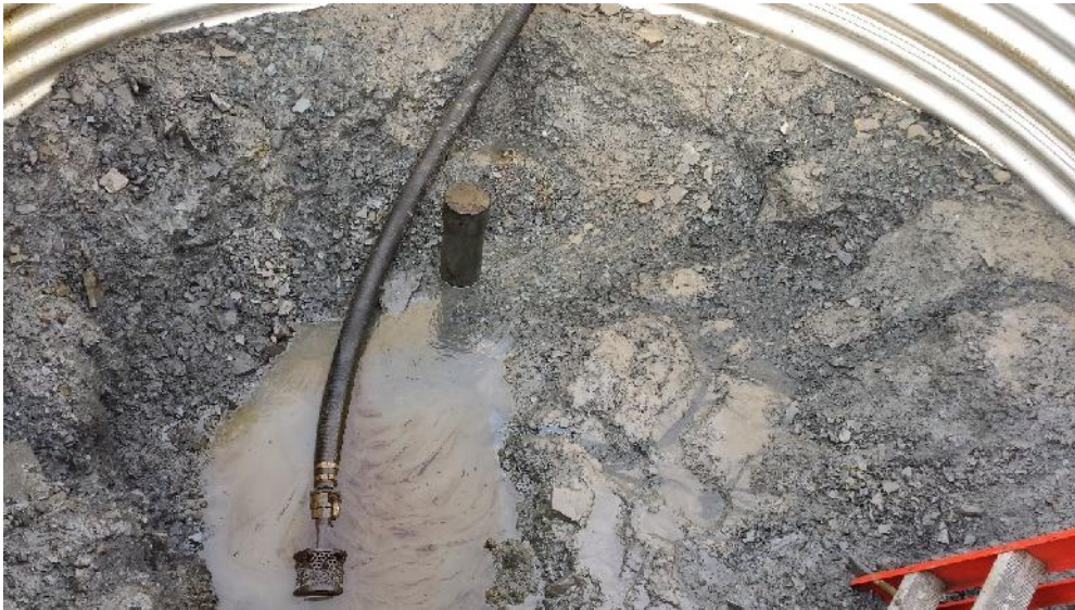
Photo 2 – Exposed well casing No.1 with existing threaded coupling attached.
