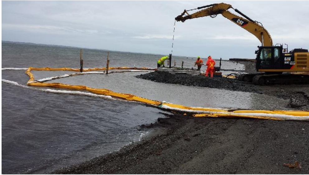
Photo 3 – View of work site at well casing No. 2.
