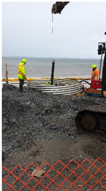
Photo 2 – Workers positioning extension pipe onto existing well casing No. 2.
