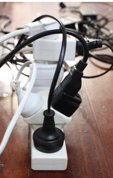
Figure 8-3 | Did you know that an overloaded power bar can get hot enough to burn?
