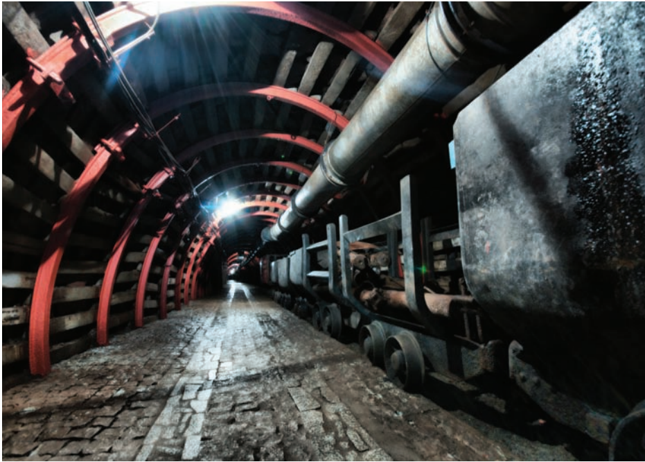
Figure 18-6 | Without proper controls, coal dust can create explosions in enclosed areas.
