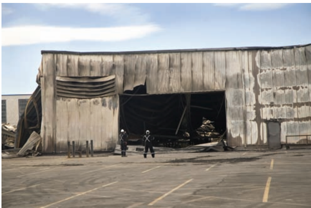
Figure 15-3 | Safety inspectors looking at the remains of a fire at a building supply site.
