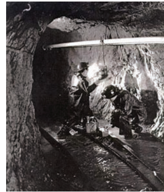
Figure 1-13 | The air quality of the underground mines posed one of the greatest threats to miners in St. Lawrence. In this image, miners are taking an air sample in the underground mine.
