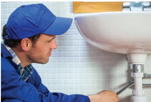
Figure 9-6 | Bump caps can resemble hard hats. Some are much more casual. But, they should never be worn as a substitute for hard hats.
