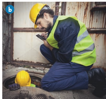
Figure 18-3 | How might confined space entry present hazards to workers a) performing a house inspection b) performing sewer maintenance
