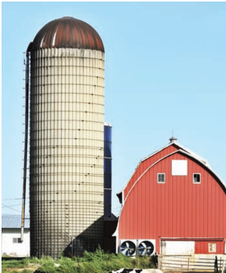
Figure 18-5 Dust explosions may occur in grain silos. Dust can arise from activities such as transporting the grains and filling the silos.
