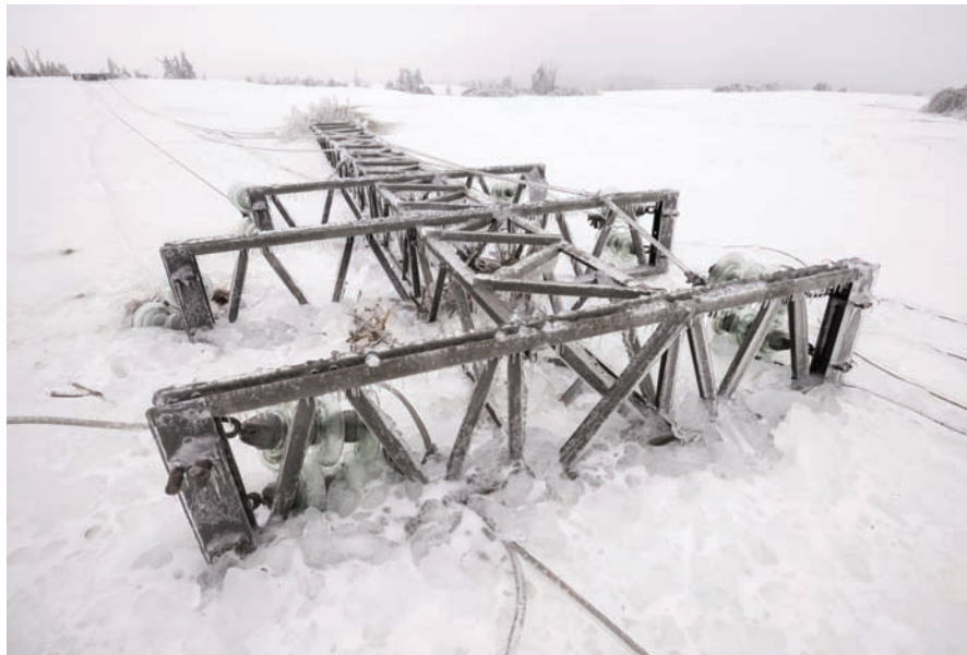
Figure 8-7 | Never approach downed power lines.
