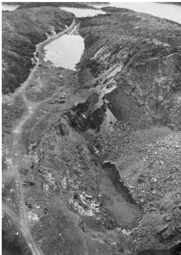
Plate 24. Aerial view looking northeast of Little Bay Mine glory-hole in the foreground (ca. 1988).
