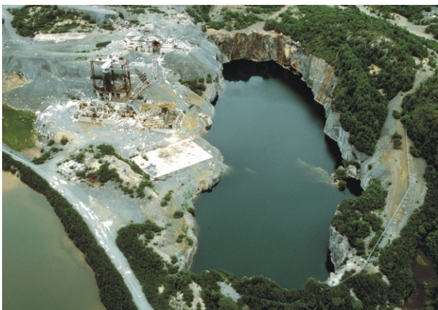
Plate 28. Whalesback Mine. Remnants of mill and headframe on left, tailings pond on extreme left, cave-in in centre (ca. 1988).
