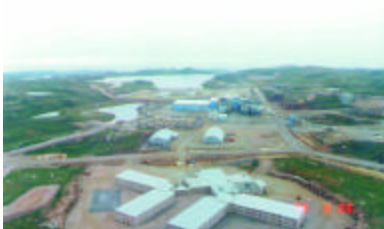
Plant Site Before Rehabilitation
