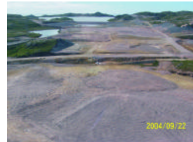
Plant Site After Rehabilitation
