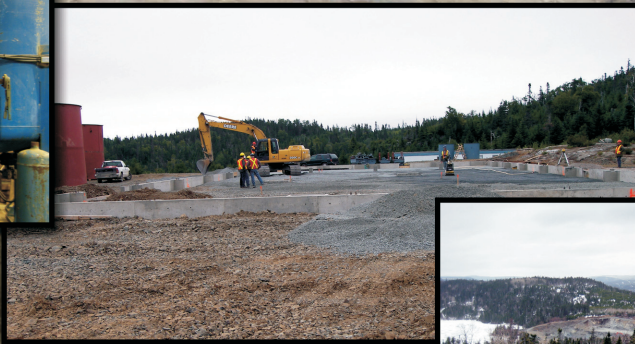
Mine Site Construction - Pine Cove
